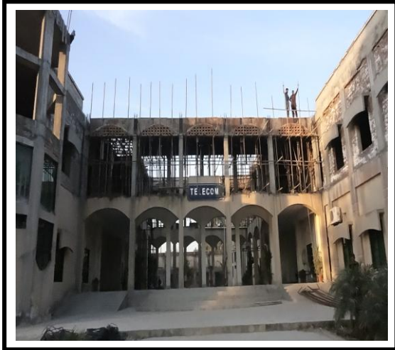
Telecom Engg Dept – 1 st Floor Cost 45.9 M
