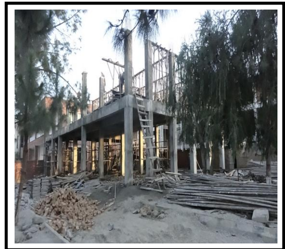
Extension of Civil Engg Dept Cost 16.5 M
