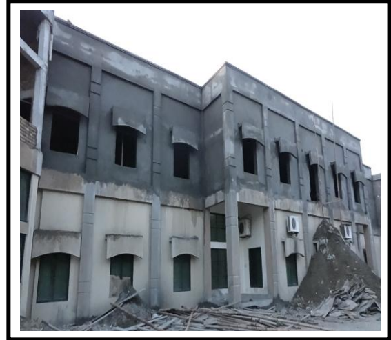
Telecom Engg Dept – 1 st Floor Cost 45.9 M
