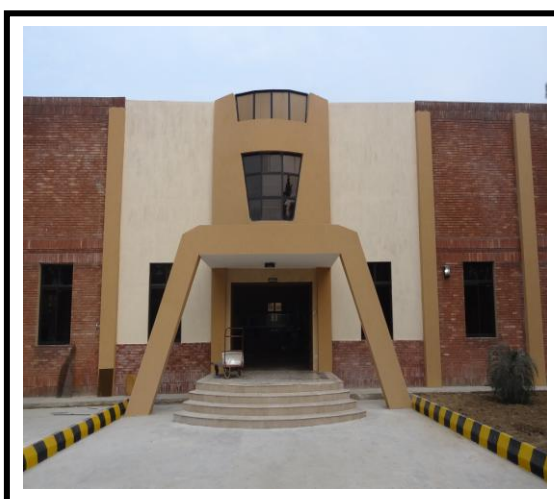
Hydraulics Lab - Cost 4.9 M
