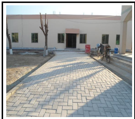
Extension of Library, Sub-Campus Chakwal – Cost 4.0 M
