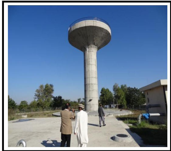
Water Tanks & Filtration Unit Cost 54.44 M
