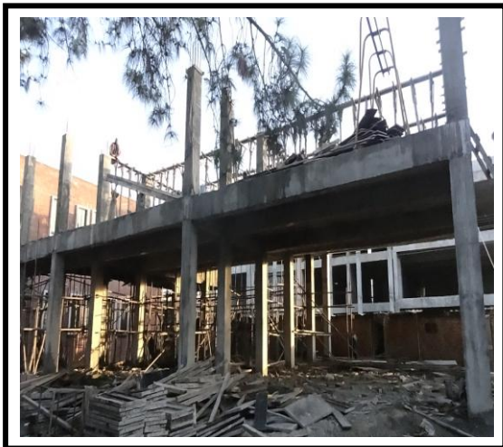
Extension of Civil Engg Dept Cost 16.5 M
