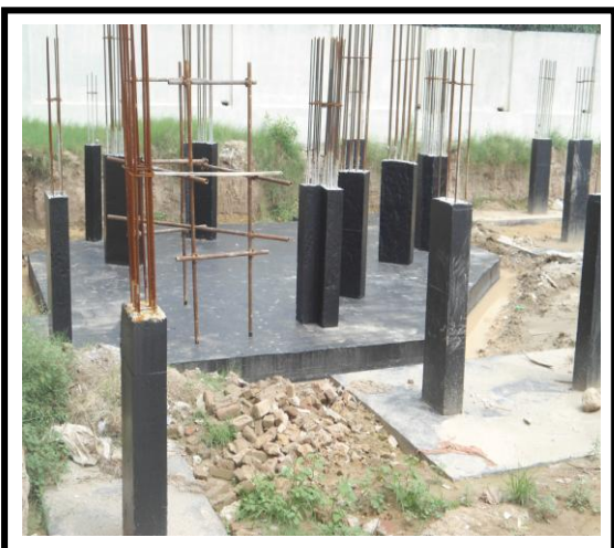
Faculty Hostel – Sub Campus Chakwal - Cost 18.7 M
